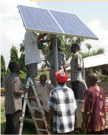
PV Water Pumping Training day in Ghana (Courtesy Geoff Stapleton, Australia)
