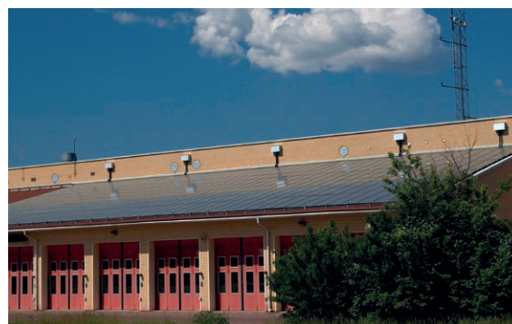
159 kW PV system on a rescue station, Falun, Sweden (Courtesy Ulf Malm, Sweden)
