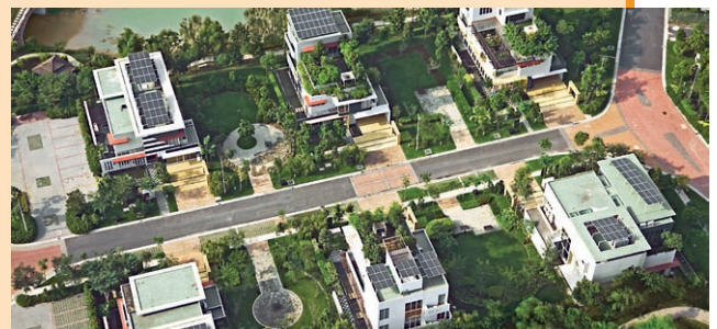
Grid connected PV systems in Malaysia (Courtesy of Ptm)
